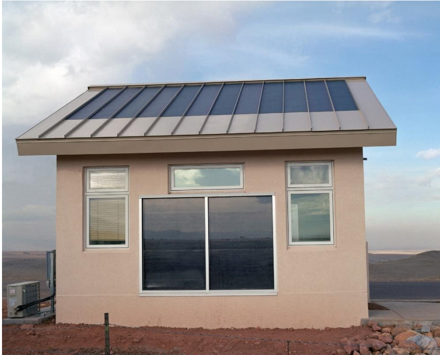
Figure 5: National Renewable Energy Laboratory: Trombe wall Image Courtesy of the US National Renewable Energy Laboratory
